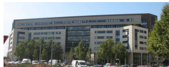
Building A view
