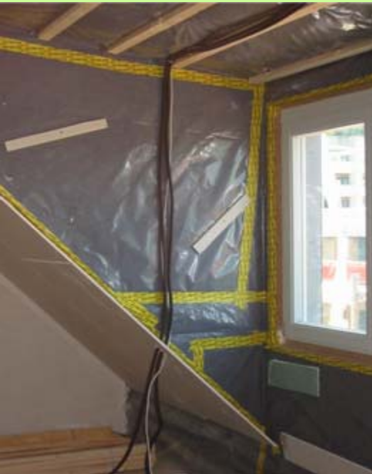
Air tightness in the attic
