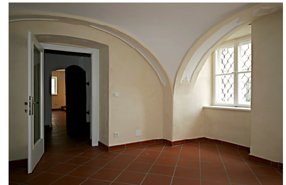
Removing the existing floor
