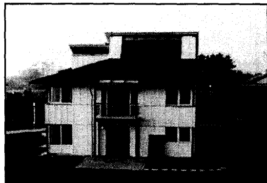
Figure 11.2 SOS Kinderdorf, Zwickau, Germany: 2.9 kW p roof-integrated PV system. Frameless architectural laminated glass with amorphous silicon cells.
