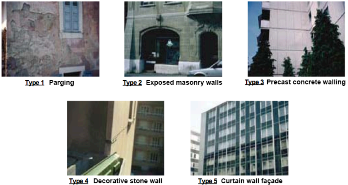
Figure 3: Illustration of the notion of « Types » - here the façades
