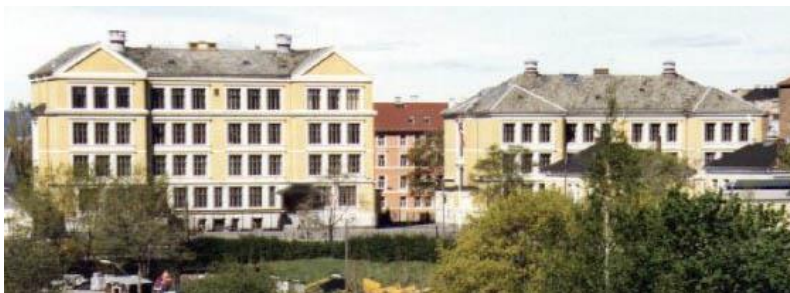
Figure 101: The east facade of the two main buildings before retrofitting.
