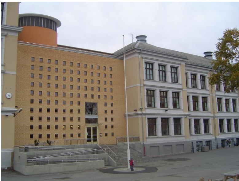
Figure 102: The east facade after retrofitting with the new connection building and new air intake at the top.
