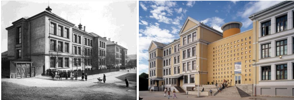
Figure 108: The east facade long before, and after renovation.
