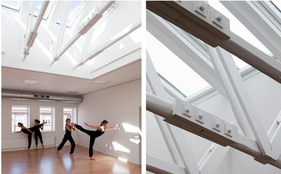
Figure 60: The roof lights provide lots of daylight to the first floor in the building.
