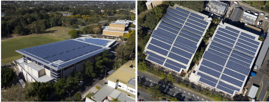
Figure 106: University of Queensland PV array, left UQ centre building, right Multi Level Carpark 1. Source: http://www.uq.edu.au/solarenergy/pv-array/st-lucia
