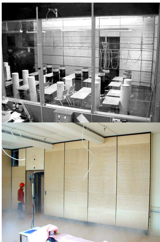
Figure 104: Smoke tests were done in laboratory (upper picture) and at site: the tests showed even distribution of supply air from the perforated wall. Maximum measured air velocity was 0.2 m/s.
