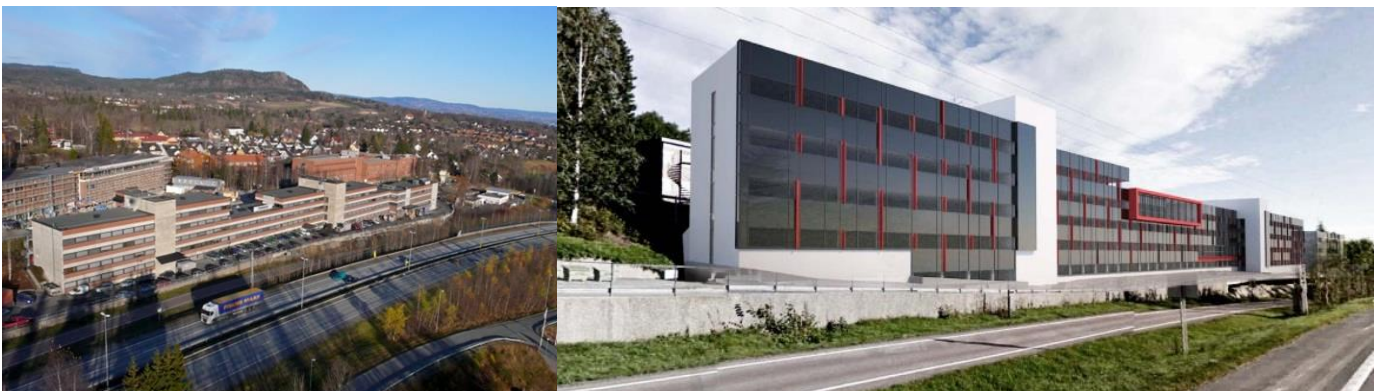
Figure 97: Solbraaveien 23 before and after refurbishment.
