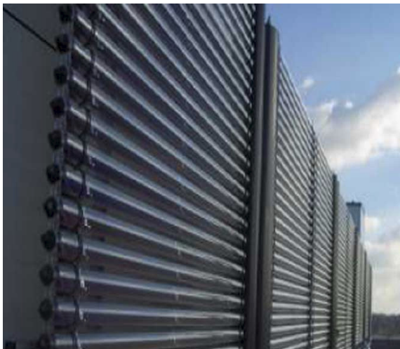
Fig. 2.7: Solar vacuum tube collector of 211 APT Sterrenveld BE (Brochure: Wouter Hilderson)
