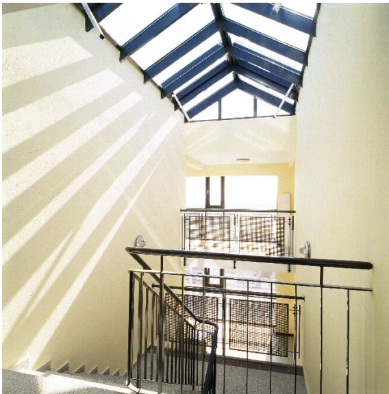
Fig. 2.14: Stair tower glazing to make this a bright, daylit space. 612 APT in Engelsby (Photos: Størmosé & Isager Architects)
