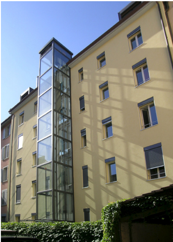
Fig. 5.5: Elevator addition in rear courtyard of 442 HIST Zurich. (Photo: D. Enz)
