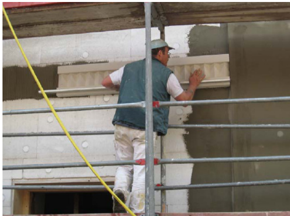
Fig. 5.1: Placing new cornices over insulation in 142 HIS Purkersdorf (Photo: Architekturburo Reinberg)
