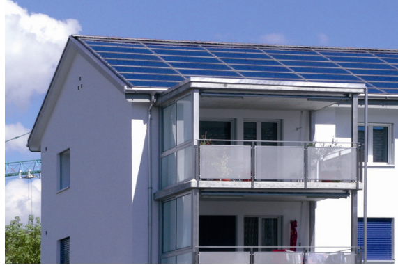
Fig. 2.8: PV Roof of 413 APT Staufen CH (Photo AEU GmbH, Wallisellen CH)
