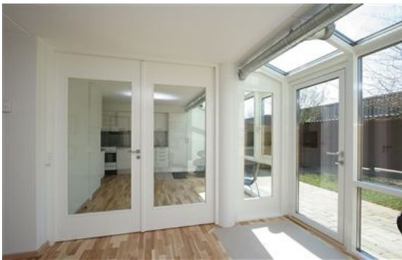
Fig. 3.3: New bay windows of 621 Alberslund DK (Photos: BoVest)
