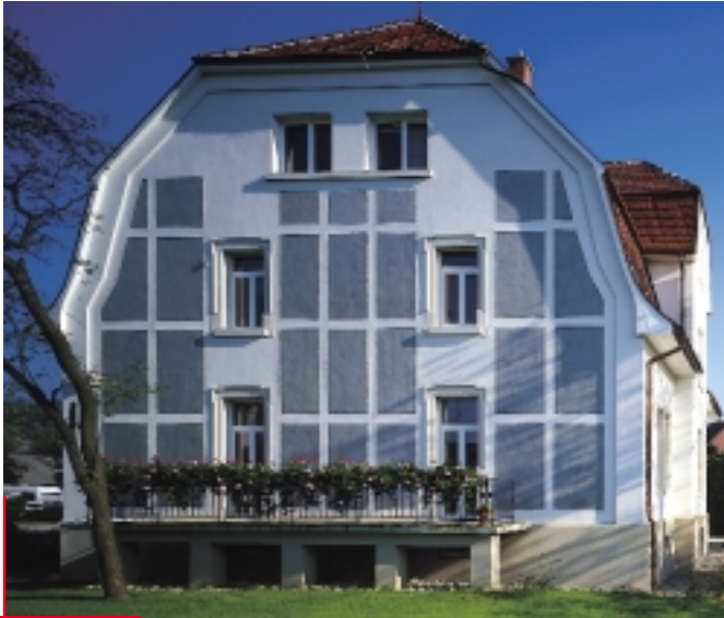
Facade with transparent insulation (Fraunhofer ISE, Germany)
