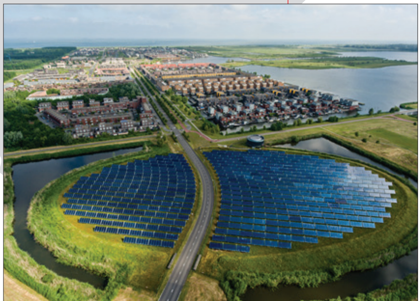
▲ The 7,000 m2 solar thermal collector field on Zoneiland Almere (Almere Solar Island) is one of the largest of its kind in the world. (Source is Nuon Vattenfall)
