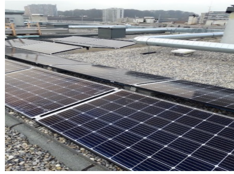
Figure 15: Solar panel installation on one of the roofs (©YellowPrint)
