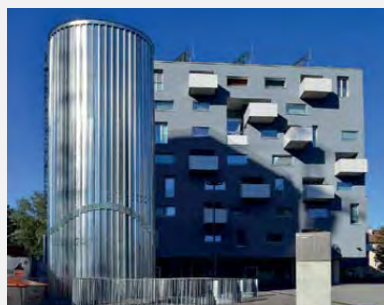
Solar assisted residential area Vallda Heberg in Kungsbacka, SE (bottom left)
