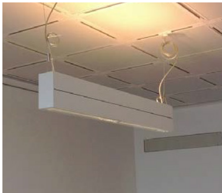
Figure 3. Luminaire with direct and indirect light output.
