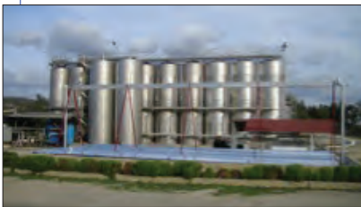
▲ Solar cooling installation at a winery in Tunisia.
