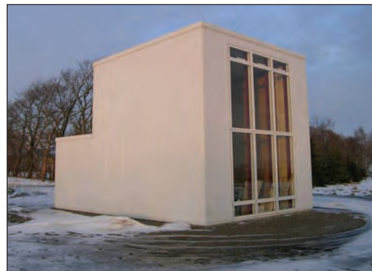
Two Task 34 test facilities: EMPA Test Cells in Duebendorf, Switzerland (on the top) and Aalborg University Double-Skin Façade Test Facility in Aalborg, Denmark (on the bottom).
