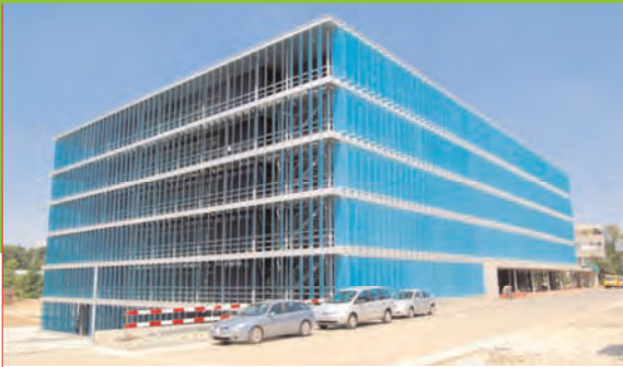
“EAWAG” research, teaching and office building in Dubendorf.
